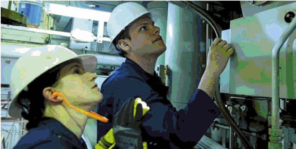
Coast Guard inspectors check out a fuel leak in a vessel's engine room. Photo: US Coast Guard
